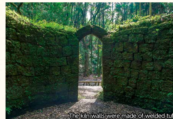
The kiln walls were made of welded tuff *The area surrounding the Terayama Charcoal Kiln is off limits due to disaster recovery work.
